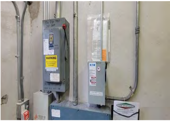
17 Elevator Disconnects
