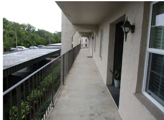
22 2nd Floor Walkway
