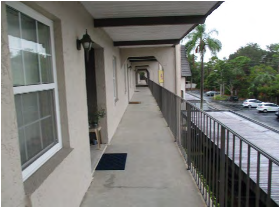
11 3rd Floor Walkway
