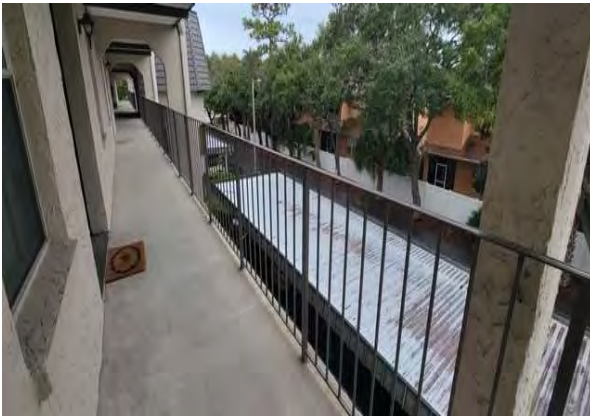
23 Walkway Railing Overview
