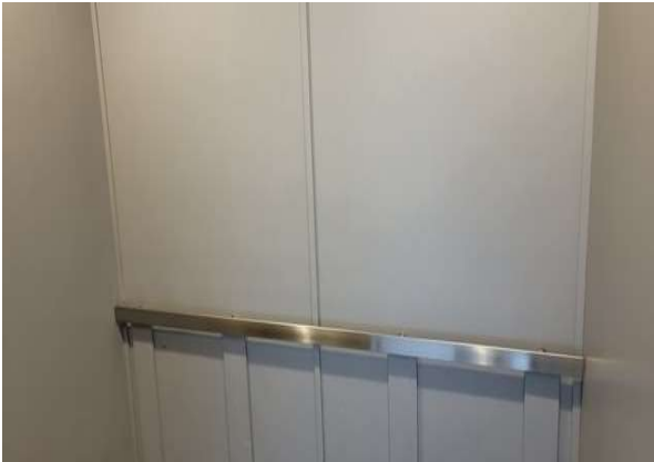
27 Elevator Cab Overview
