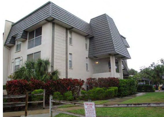
4 Left Side of Building 8765
