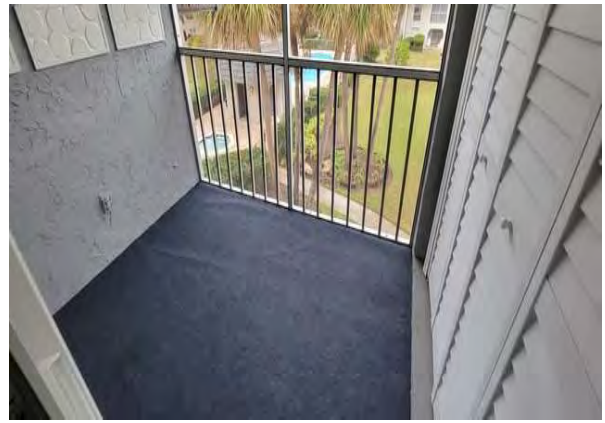
10 Unit 304 Balcony Overview
