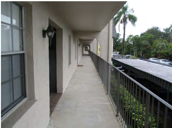
21 2nd Floor Walkway
