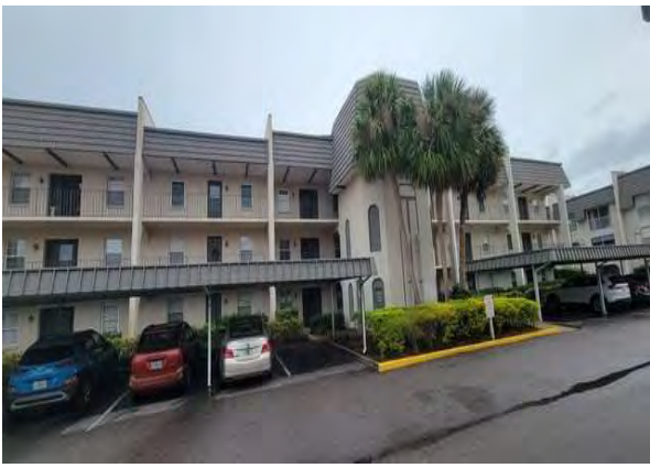
1 Front of Building 8703
