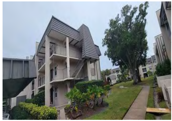
2 Right Side of Building
