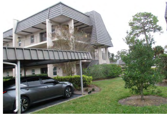
2 Right Side of Building 8765
