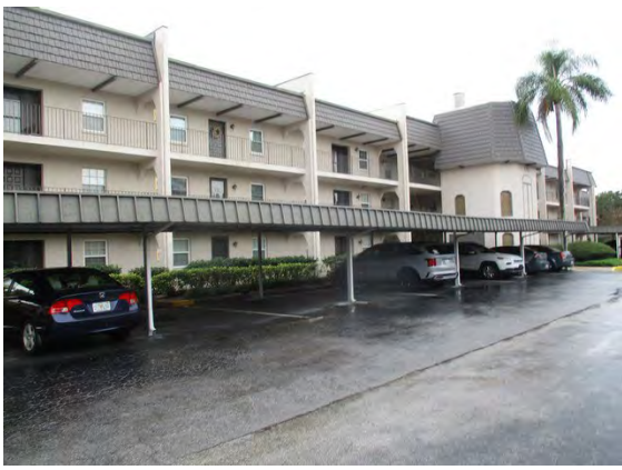
1 Front of Building 8765
