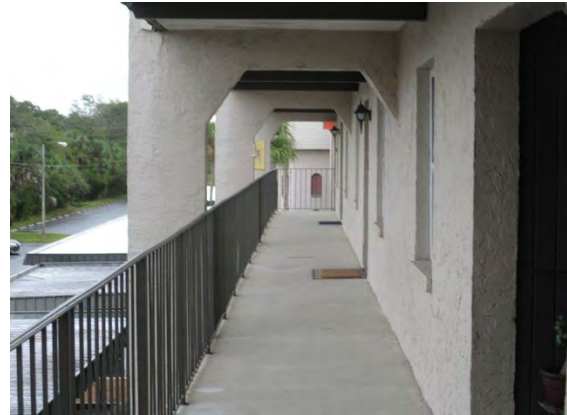
12 3rd Floor Walkway
