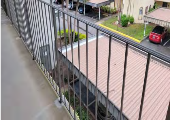
27 Walkway Railing Overview
