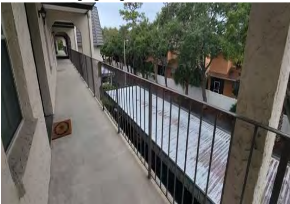
23 Walkway Railing Overview
