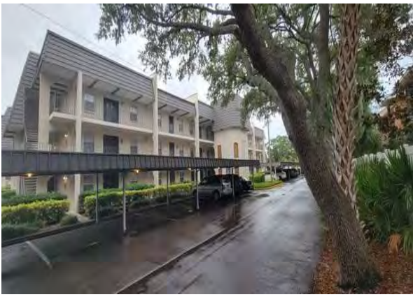
1 Front of Building 8799
