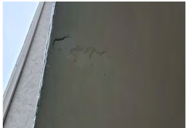
56 Cracked Walk Near Unit 106
