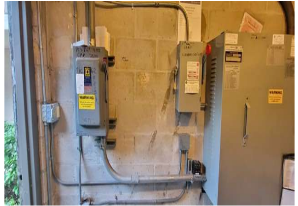
12 Elevator Disconnects
