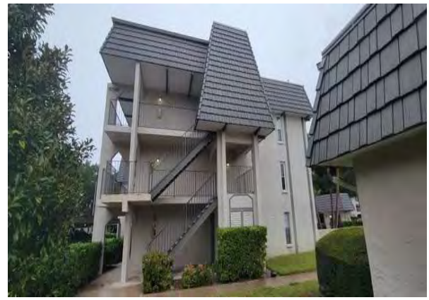
2 Right Side of Building
