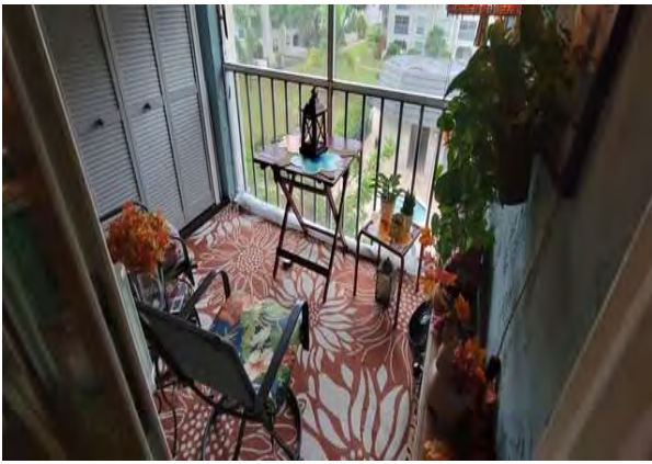
9 Unit 305 Balcony Overview
