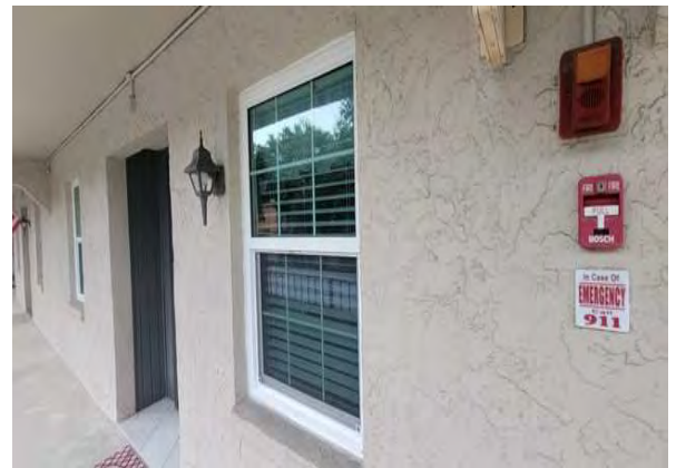
30 Unit Window Overview
